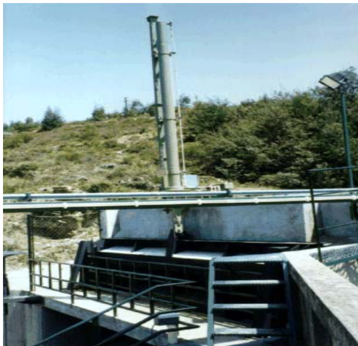
Photo 5.12: Hydraulic Cylinder
