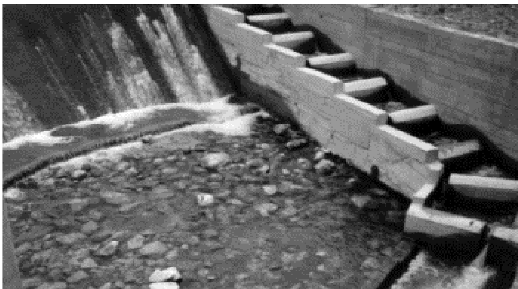
Photo 7.14: Fishpass with vertical slots
