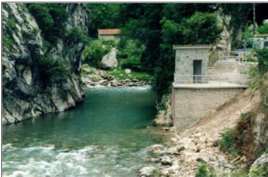
Photo 3-1 Gauging station in a river
