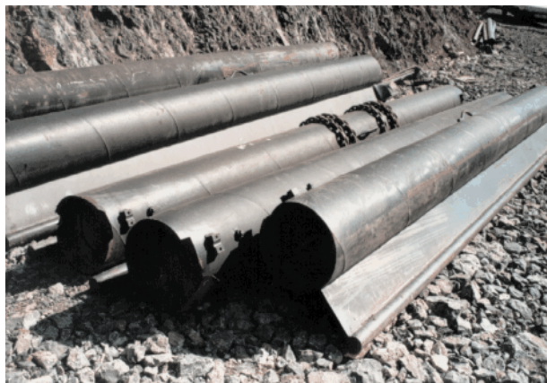
Photo 5.9: Prefabricated booms
