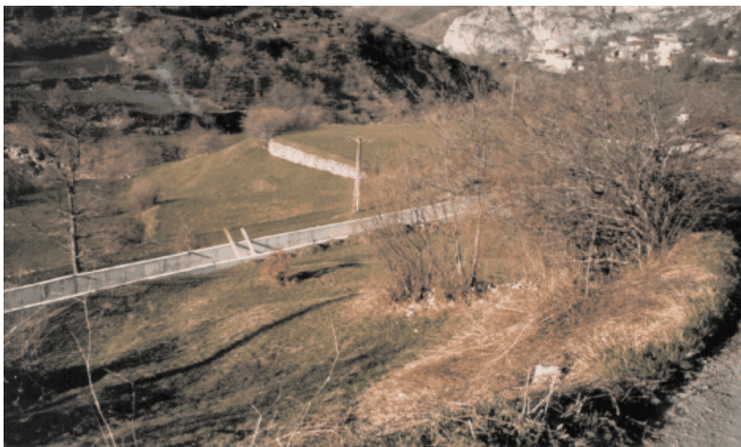
Photo 7.6: Construction phase – concrete canal
