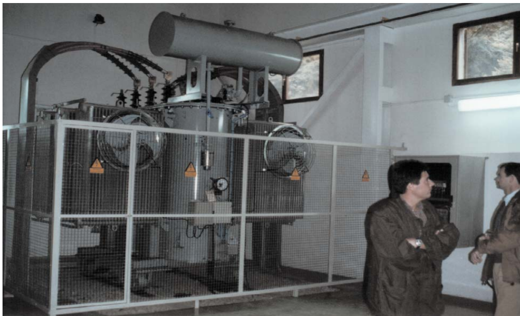
Photo 7.11: Substation located in Powerhouse
