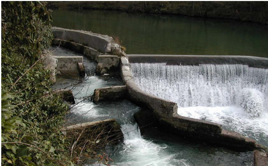
Photo 7.13: Fishpass of rustic construction
