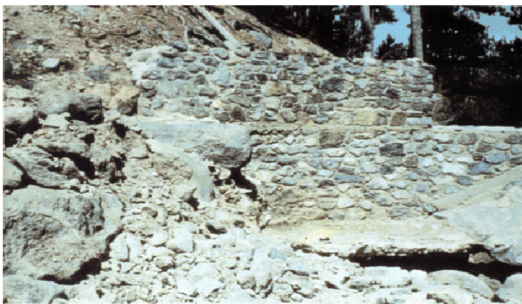
Photo 4-11 Weir undermined by seepage
