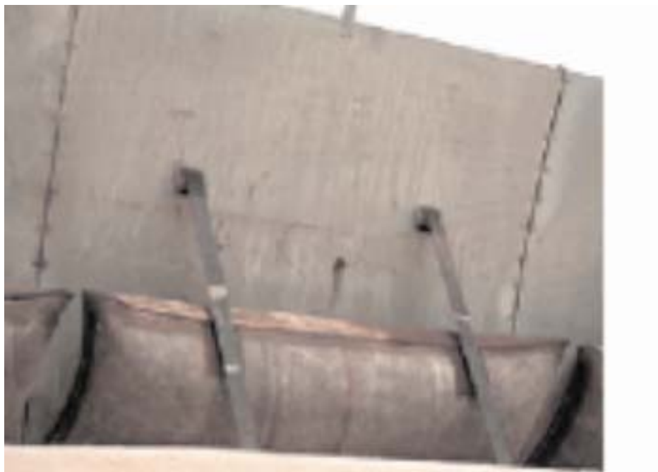
Photo 5.6: Flashboard controlled by inflatable rubber bladder
