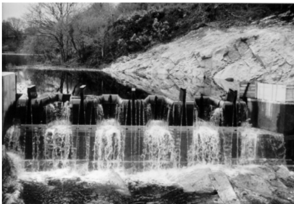
Photo 5.7: Hydroplus fusegates
