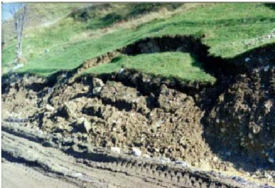
Photo 4-2 Local instabilities generated during the excavation works
